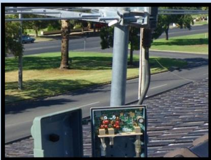
If signal is still low then a masthead amplifier can be used. This amplifier is housed in a weatherproof box and is attached to the mast just below the antenna. The reason for this is that in order to maintain signal quality, it is desirable to have minimal unwanted noise being amplified along with the TV signal.
